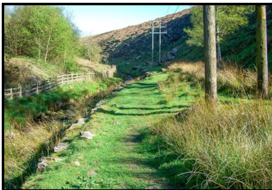
The remains of the 1812 Turnpike close to the Heathy Lea Brook It was subject to landslides and flooding. 1816 Turnpike Baslow to Owler Bar
